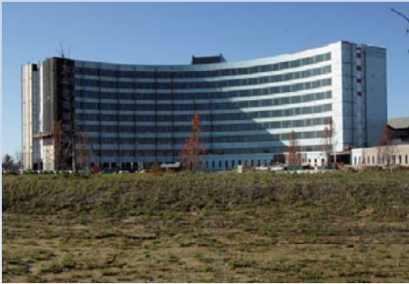
A shot of the bed tower from across the retention pond.
