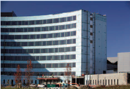
Construction continues on the bed tower.
