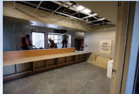
Crews work on the collaboration hub on the ninth floor.
