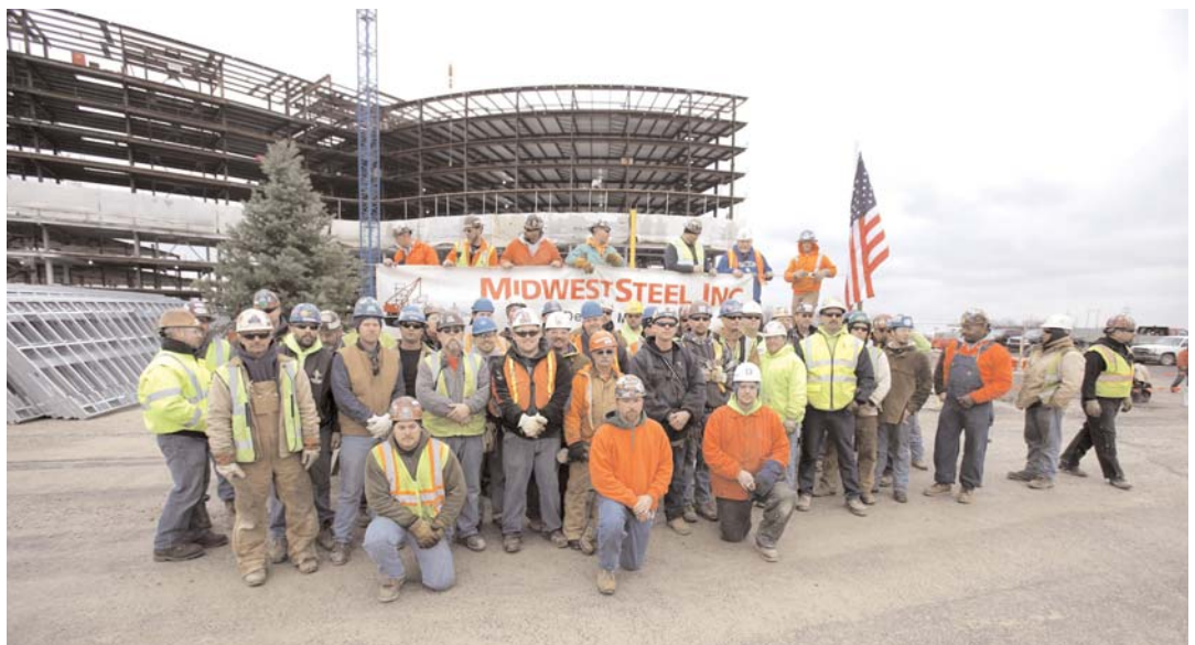
Steel workers become part of history as they pose for a photograph in front of the highest beam to be placed in the new hospital.
