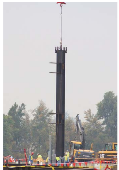
These two pictures show the first beam of steel being installed at the new hospital site between Pleasant Valley Rd. and Daniels Ln. The first piece weighed in at 20,000 pounds and was erected just after 9:00 Wednesday morning. If you'd like to watch the first piece of steel being set, become a fan of Owensboro Medical Health System on facebook.
